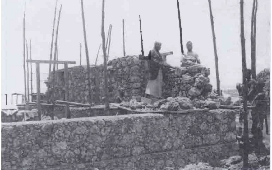
Fig. 3: Erection of mass brickwork of coral rag, Source: Archive of the Leipzig Institute for Regional Geography.
